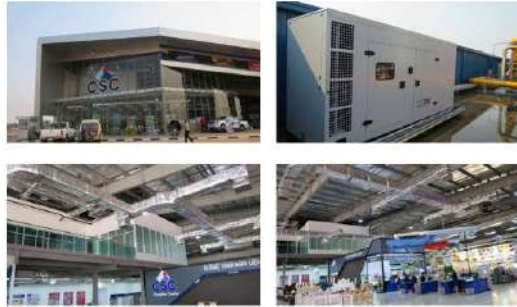
Design and Install Air-Conditioning System Water Cooled Chiller 206.9 Ton(2)
