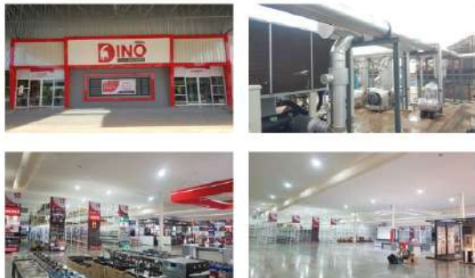
Design and Install Air-Conditioning System Air Cooled Chiller 180 Ton
